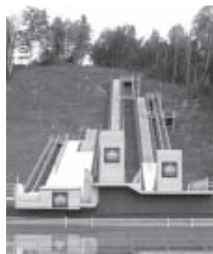
Ramps from below
