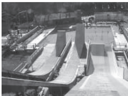
Ramps from above
